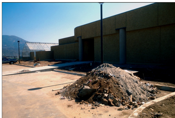
Front of OH building during construction, circa 1979
