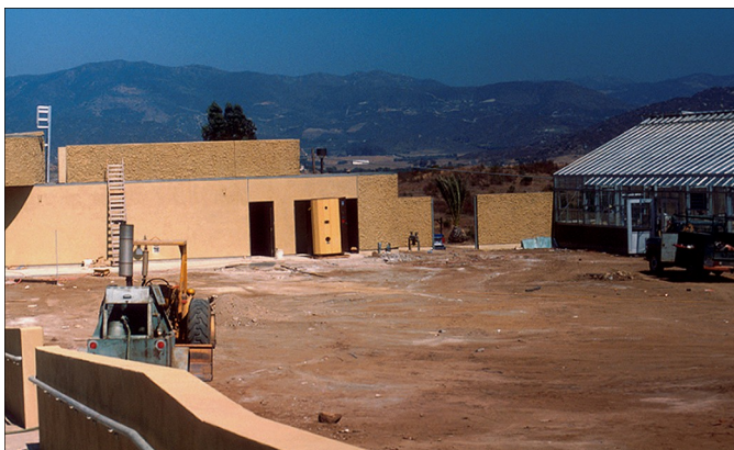
Site of the Cuyamaca College OH Department during construction, circa 1979
